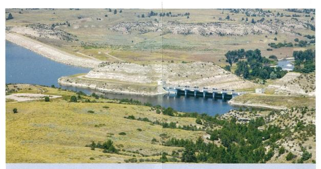
Located 11 miles east of Laramie River, the 104,000 acre-foot Grayrocks Reservoir is the principal water source for the plant. Along with other groundwater sources, it provides up to 23,250 acre-feet of water annually to Laramie River for steam production and cooling. The reservoir, which is about eight miles long, includes recreational facilities and a visitor overlook. Several species of game fish are stocked in the reservoir.
