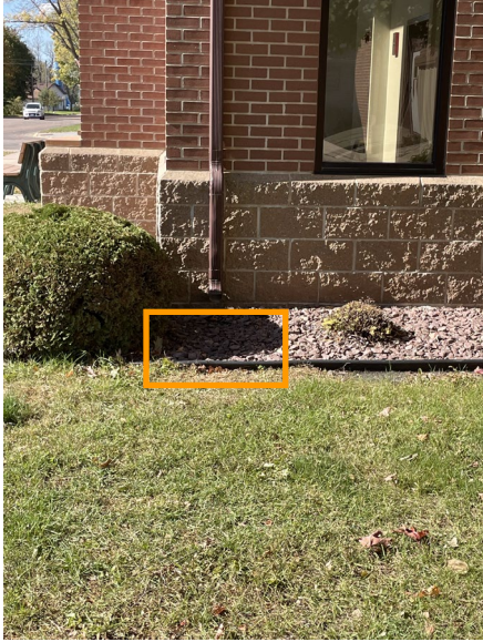
Photo 8: City to provide downspout extension at various locations, extend beyond stone (not part of project)
