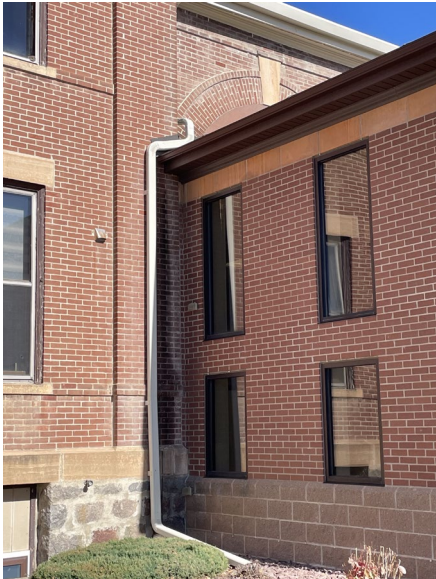
Photo 7: Monitor downspout for adequate drainage
