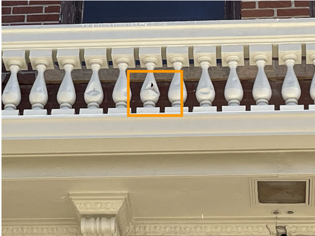
Photo 3: Repair balustrade
