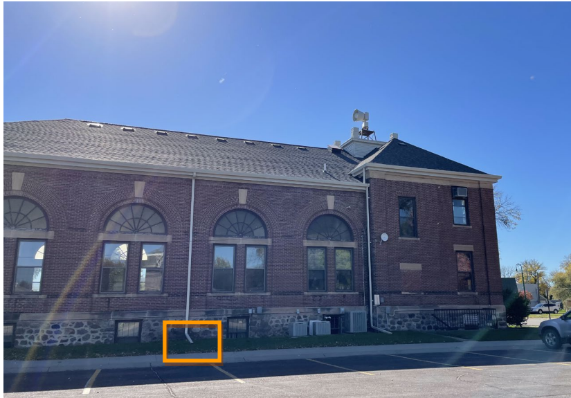
Photo 1: Alter downspouts to be removed during mowing, all locations
