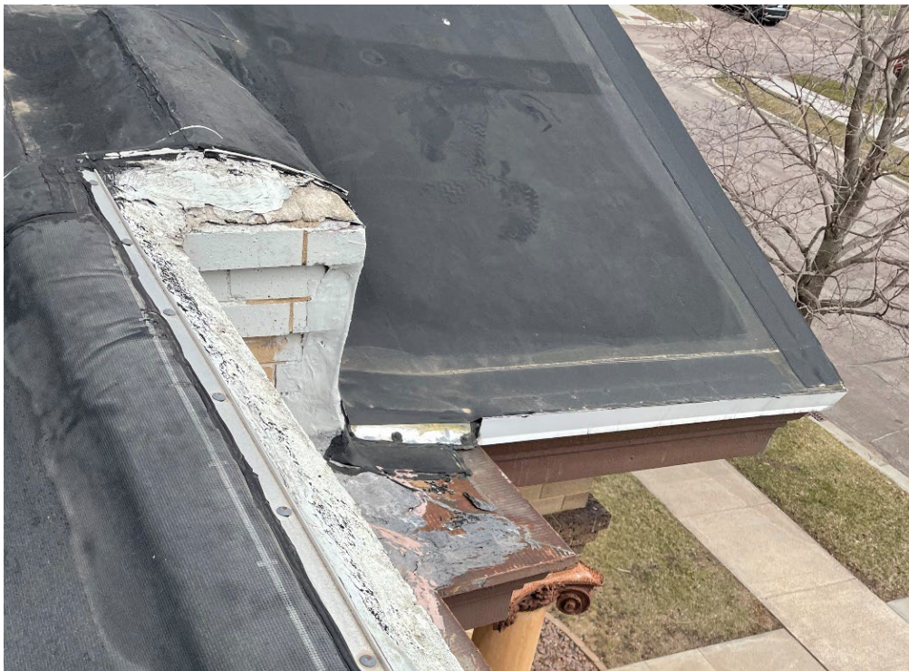
Photo No. 6: Top of east parapet with EPDM and concrete parging and roofing compound.
