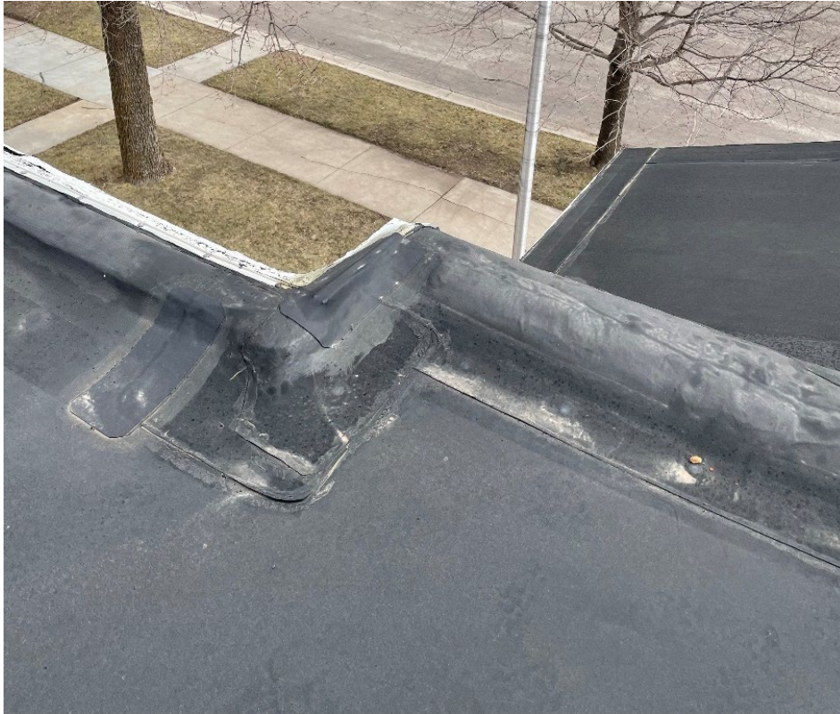
Photo No.7: Top of east parapet with EPDM and termination bar.
