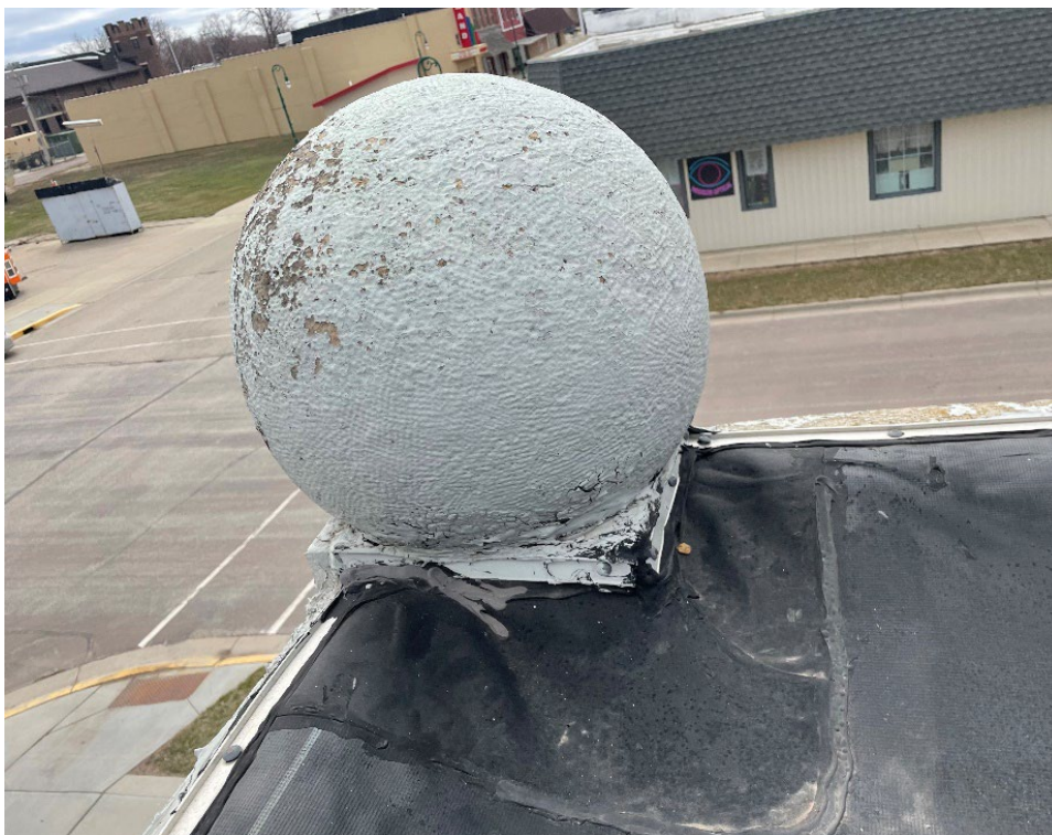
Photo No. 8: Stone corner spheres, no work to sphere, new flashing and coping for cleaner appearance.
