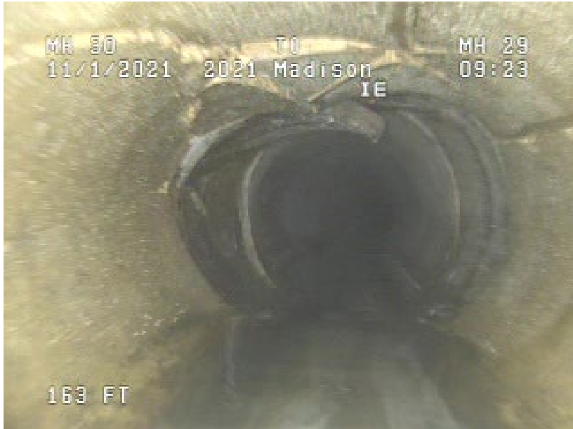
Severe Cracking
