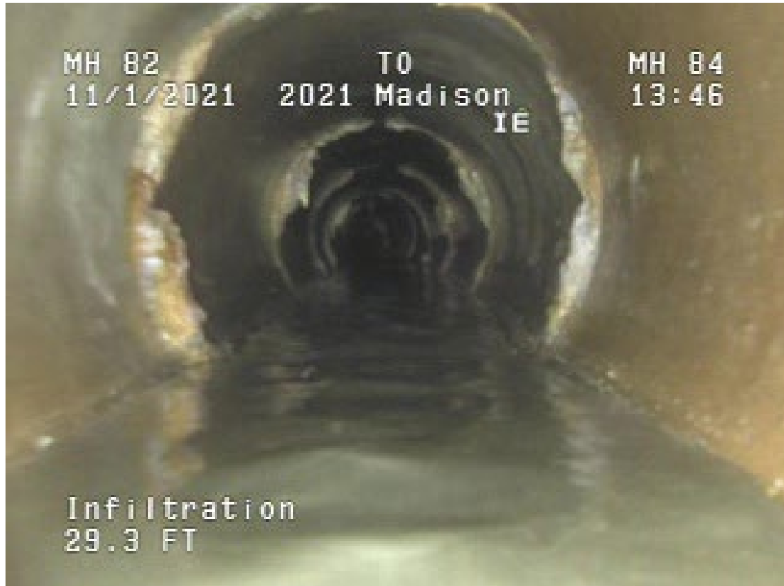
Mineral Deposits (Infiltration)
