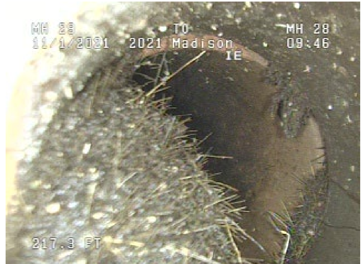
Root Intrusion at Service
