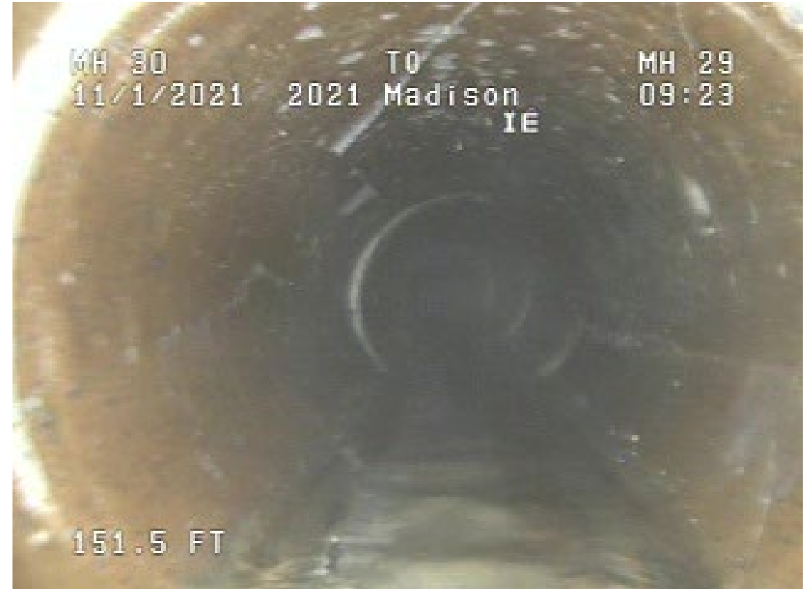
Typical Cracking
