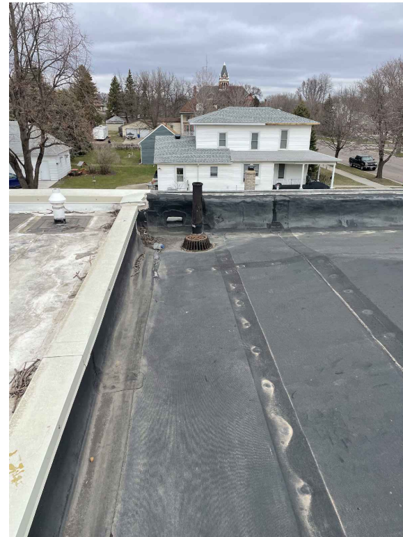
5 | Looking north. Roofs joining.
