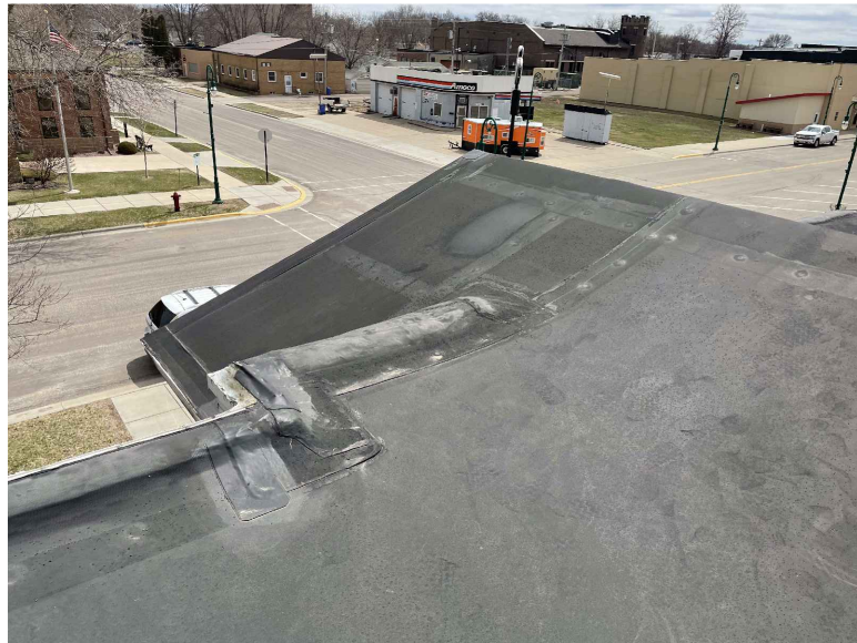
2 | Looking east. Original roof.
