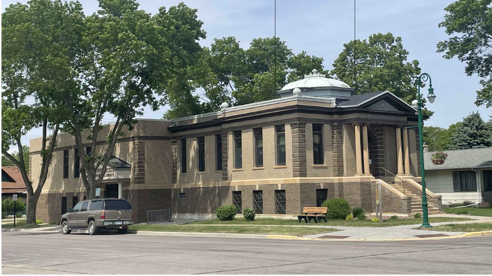
1 | Looking northwest. South Elevation and East (Front) Elevation.
