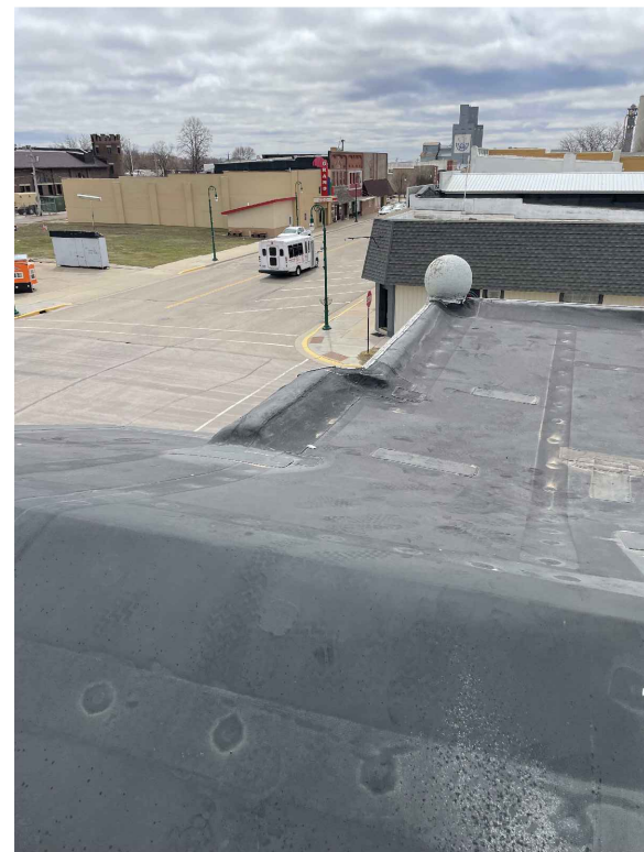
4 | Looking south. Original roof.
