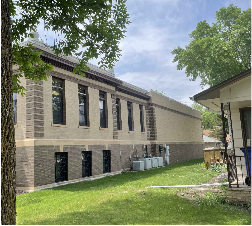
2 | Looking southwest. North Elevation.
