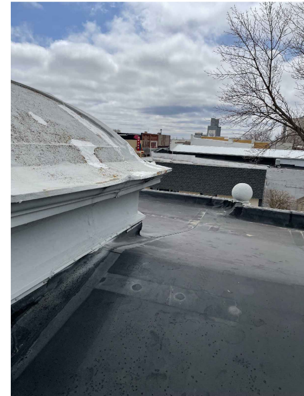
7 | Looking south. Original roof & dome.
