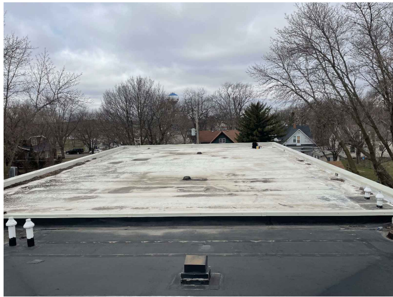
1 | Looking west. Addition roof.
